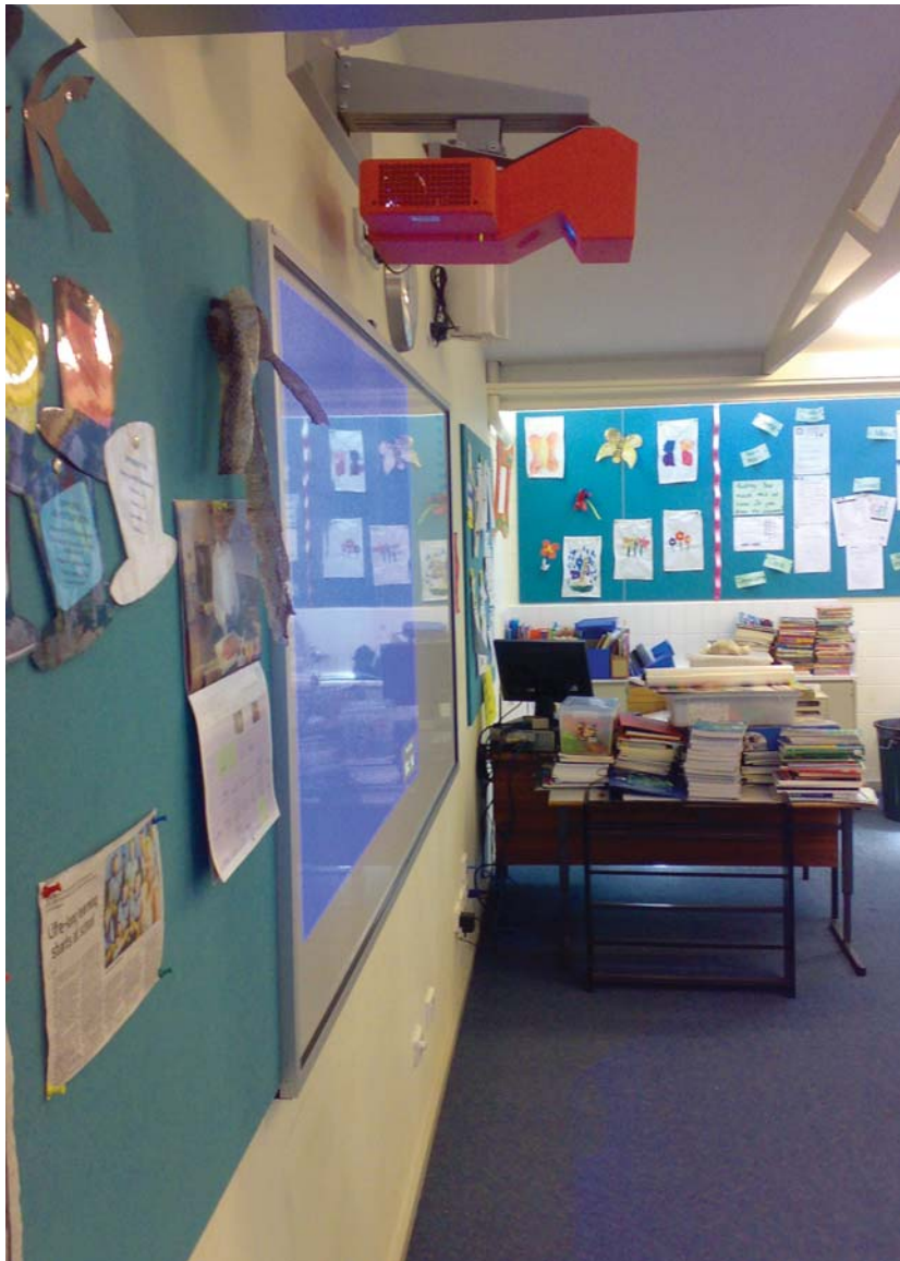
Installation in Junior School room, with 2Touch Interactive Whiteboard and side view of Sanyo's PLCXE50 Ultra Short Throw projector
