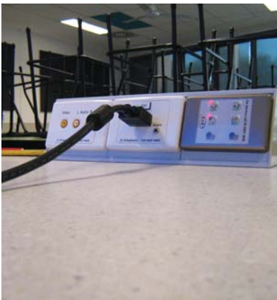
Moduline angled bench mount installed onto Science room's island bench for convenient and quick teacher access
