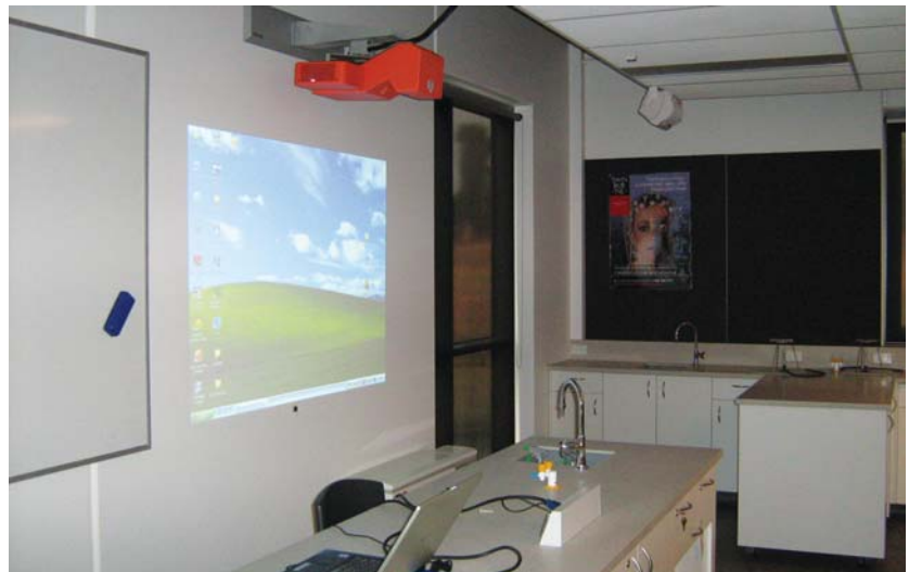
Ultra short throw projector in Psychology room can project an 80" diagonal 4:3 image in XGA resolution from an 8cm throw distance
