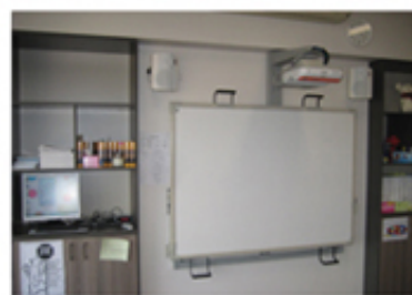
Classroom Installation - Korowa Anglican Girls School
